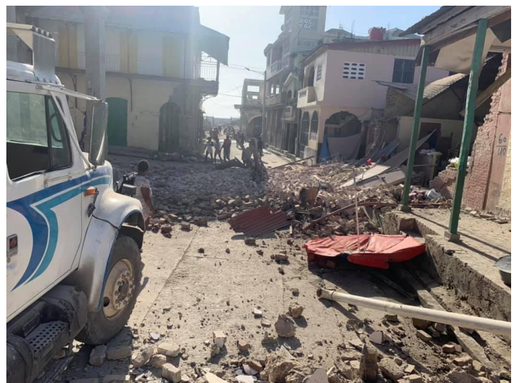
Damage to Downtown Jérémie
